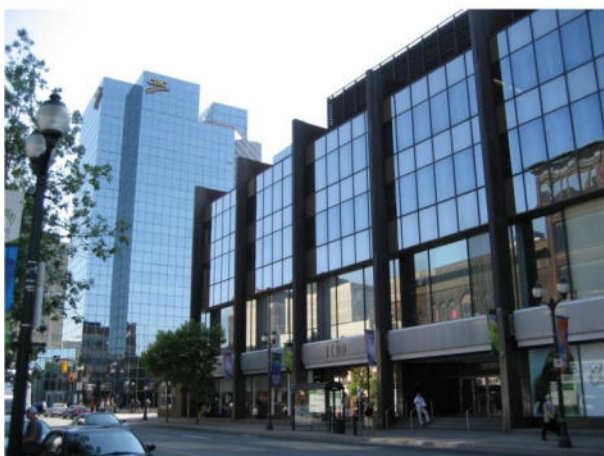
Lloyd D. Jackson Square (Mall), Commerce Place Complex
